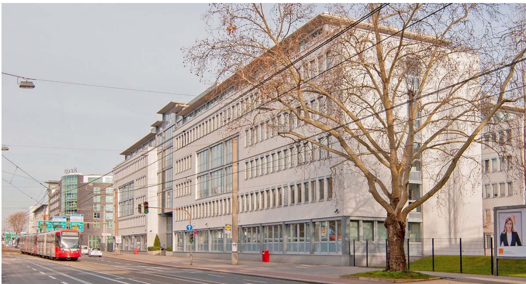
Von-Gablenz-Strasse 2-6 © Greif & Contzen 2019
