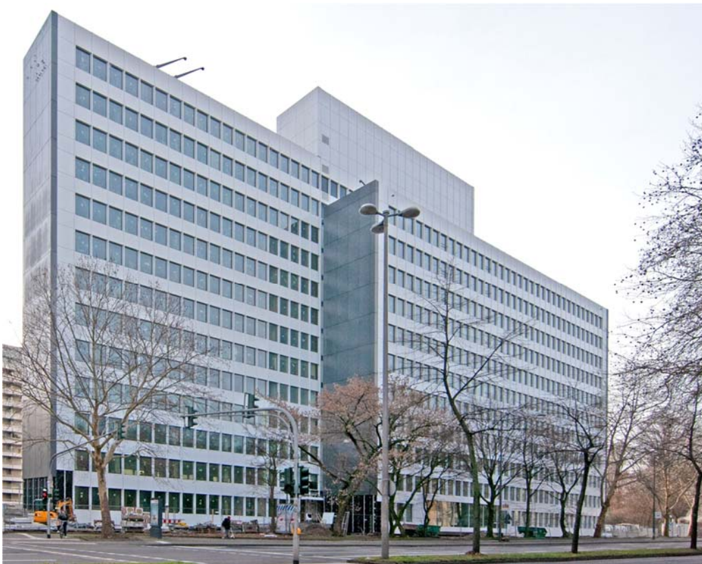
Soon to be completed: "One Cologne" on Innere Kanalstrasse © Greif & Contzen 2019
