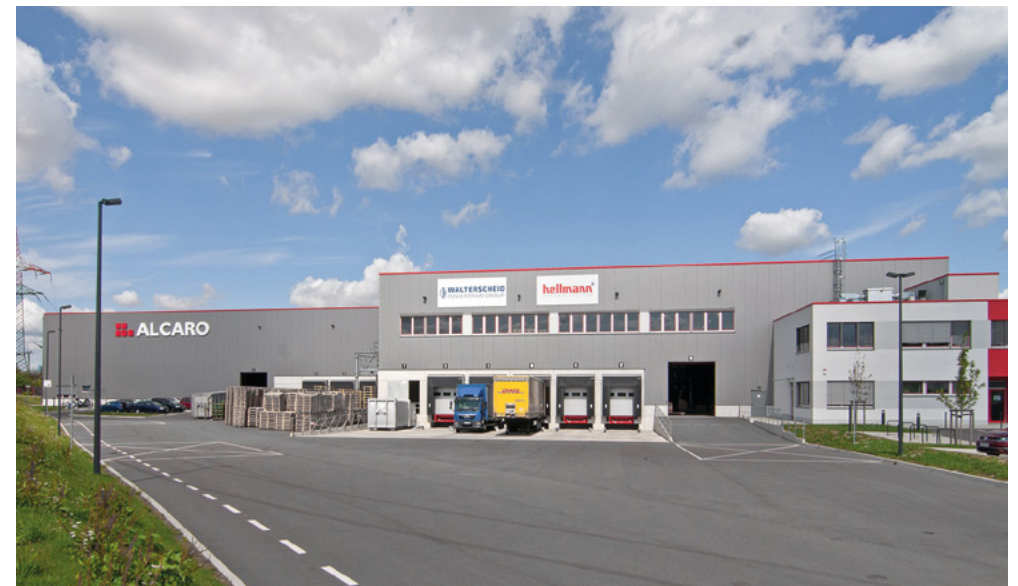
Building extension of a logistics centre in Kerpen
