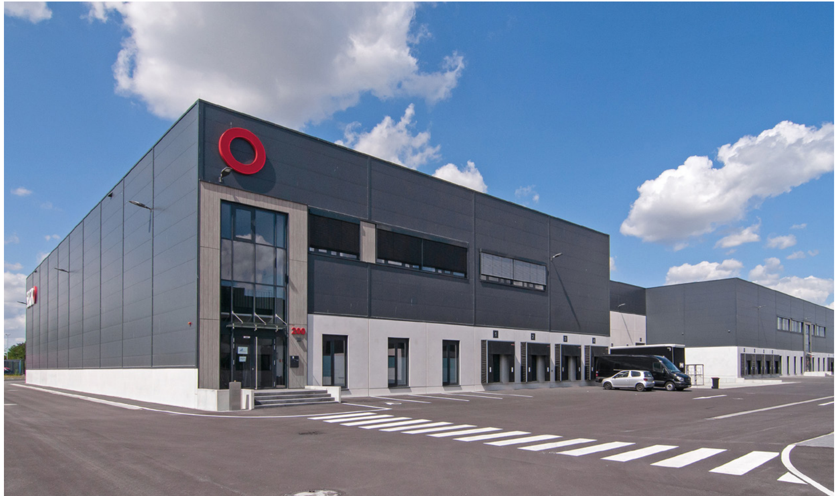
Part of the new commercial estate in Cologne-Bickendorf
