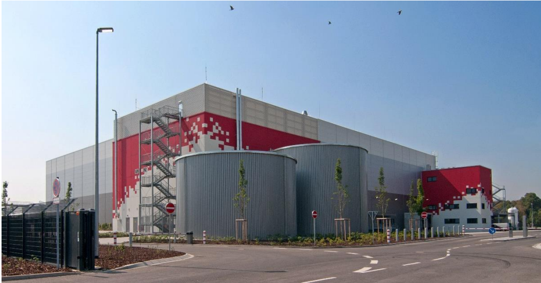
New building in Cologne Niehl © Greif & Contzen 2018
