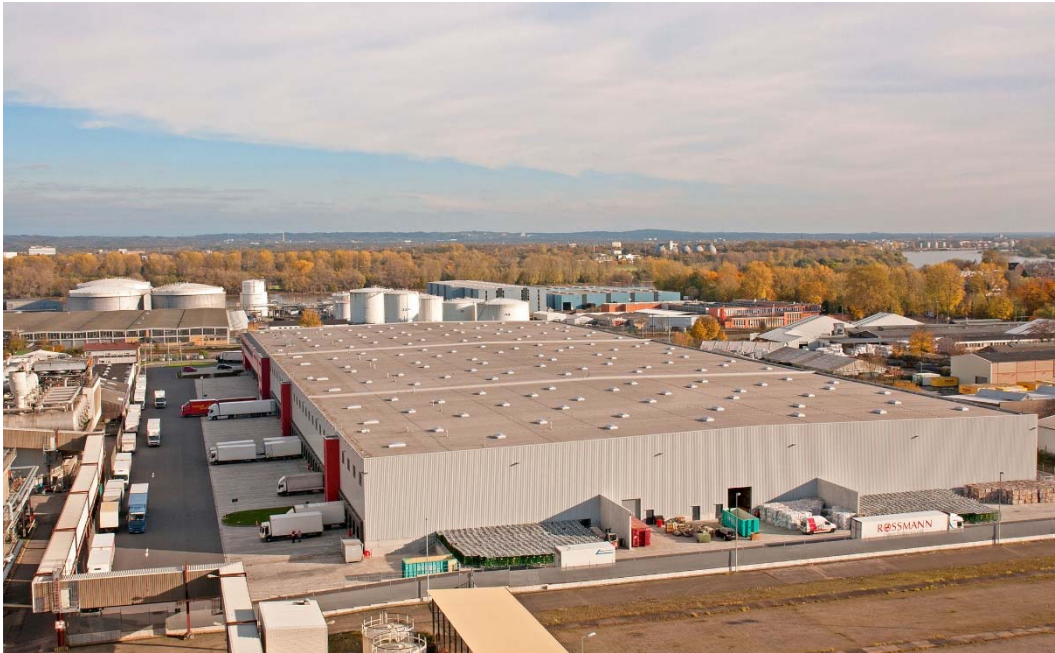
Emdener Straße © Greif & Contzen 2016
